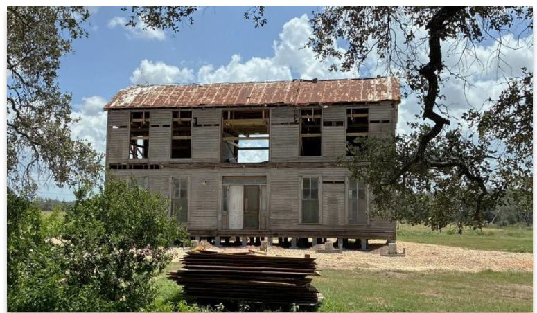
Bottom right: The large two-story portion of the house as it sits with roof sections newly reattached.
