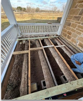
Front Porch Restoration
